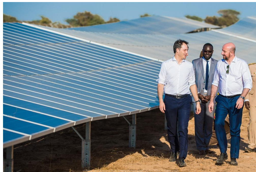
Figure 3. The El Carmen solar plant in El Salvador (Left)
